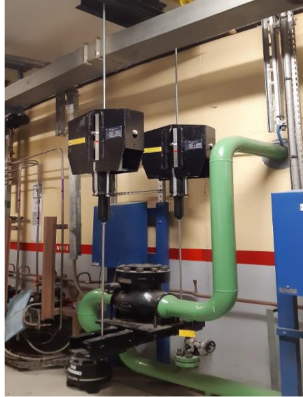
Renforcements tuyauteries ASG
